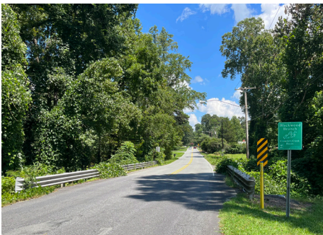
9. Bridge on Linwood Road over Blackwood Creek
