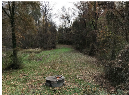
10. Sewer easement along Blackwood Creek, south from Linwood Road
