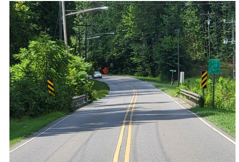
4. Bridge on Archie Whitesides Road over Crowders Creek
